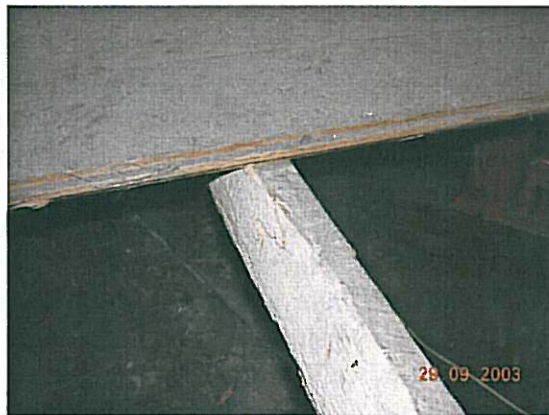
Lyctus Borer damage to floor joists
