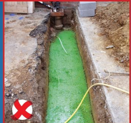
Filled with chemicals and back-filled
