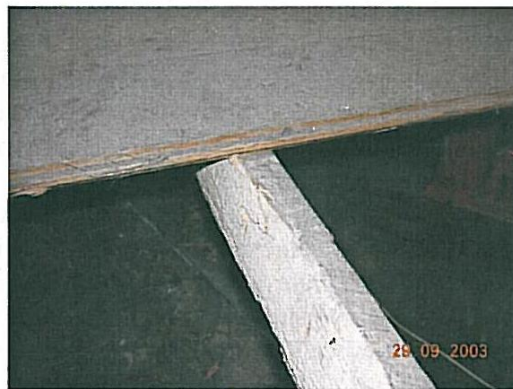
Lyctus borer damage to floor joists
