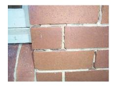
These pictures illustrate the damage by Mortar Bees, the have excavated the mortar from the joints of the bricks.
