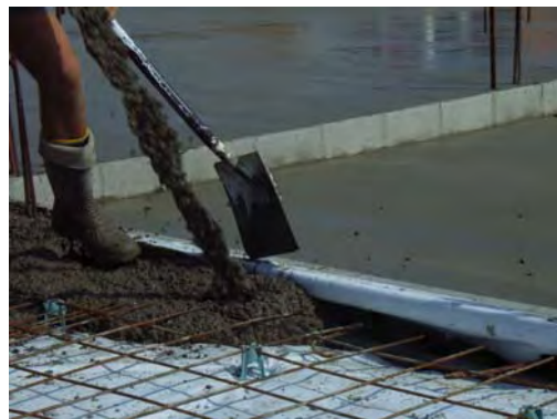
Pouring of slab into Door Sill Block.
