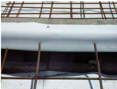
Rear view of Door Sill Block after installation of HomeGuard
