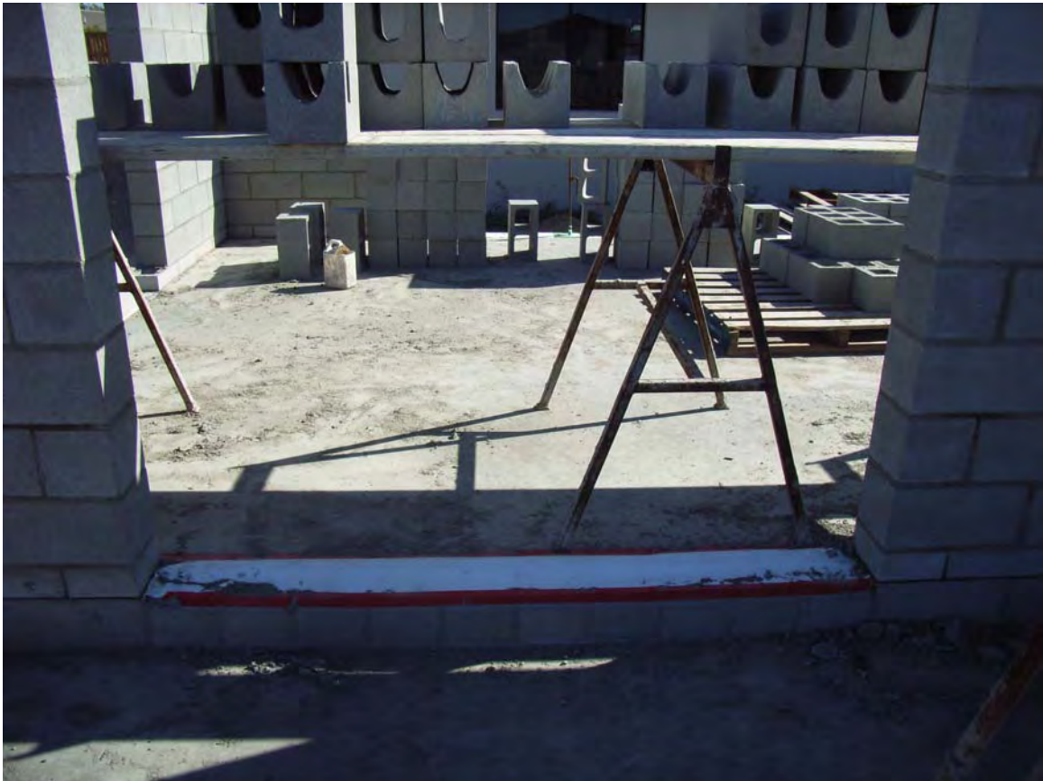
Typical Block construction showing HomeGuard installation at the step down
