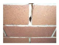
It would appear the when the Mortar Bee attack is advanced then the natural erosion of mortar from the brick joints in the immediate area will also increase.
