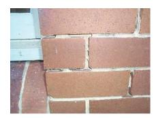
These pictures illustrate the damage by Mortar Bees, the have excavated the mortar from the joints of the bricks.
